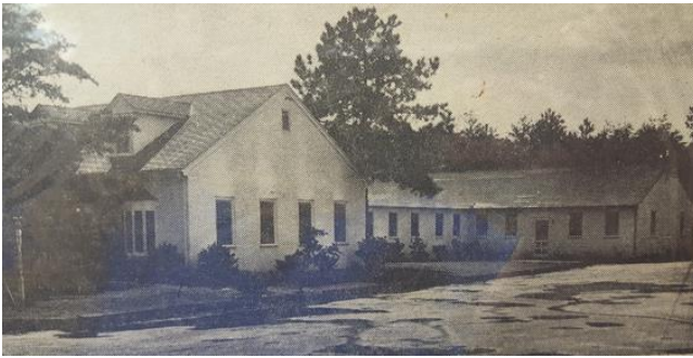
New addition completion
